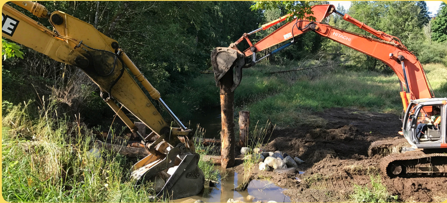
We are lucky to work with fantastic contractors on our projects. Wrangling 50' long logs is a big job, but the excavator operators with RV Inc. are more than capable. Pictured above is the second instream log jam installation at the Lower McLane restoration site.
