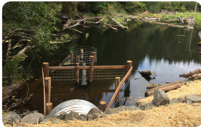
Upstream of the newly installed culvert, SPSSEG also installed a beaver deceiver. We love our beavers, but they do have a habit of incorporating fish passable culverts into their dams.
