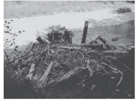
Completed log jam after two years.
