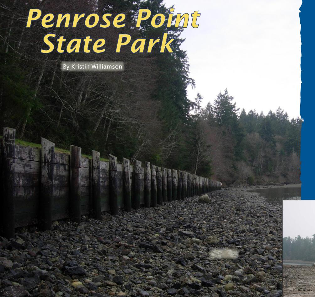
Work to remove a large, 700 foot long creosote treated bulkhead and rip rap armor has begun! Heavy equipment was mobilized to Penrose Point State Park on January 15th 2013 to begin the difficult task of dismantling and hauling away this old, failing bulkhead
