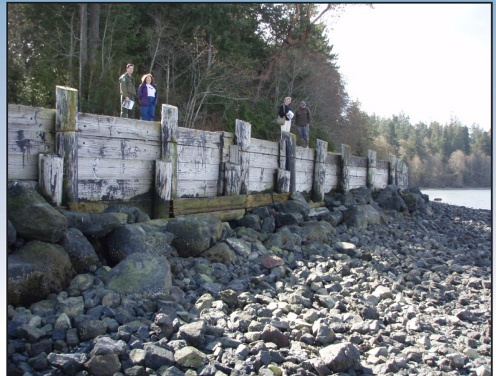
Penrose Point Bulkhead
