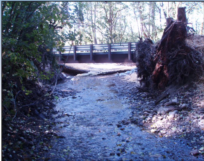
Powell Creek Culvert Replacement
