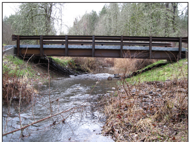
Lackamas Creek - Post-project
