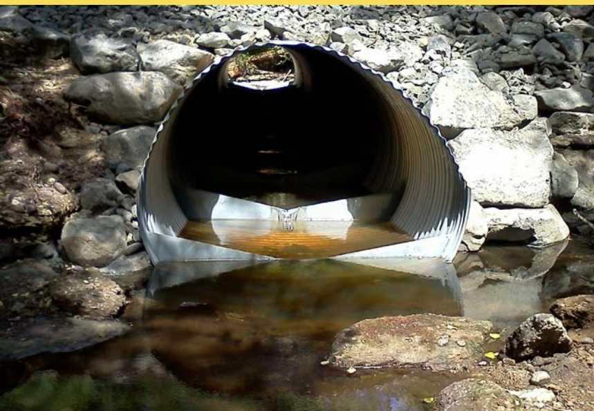
Below: Installed fishway style culvert
