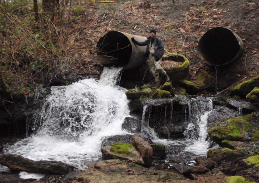
Above: Perched dual pipe culverts
