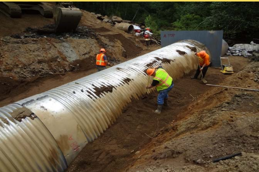
Above: New nine-foot fishway culvert being installed
