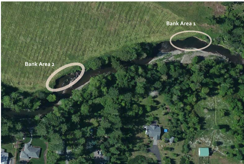
Figure 6: Eroded bank areas within project boundaries. Bank erosion was observed to be rapid in bank area 2.
