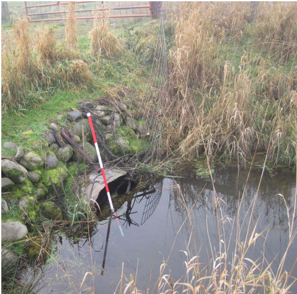
Figure 1: Outlet channel culvert to be removed within wetland rehabilitation area. Photo taken December 11, 2013.
