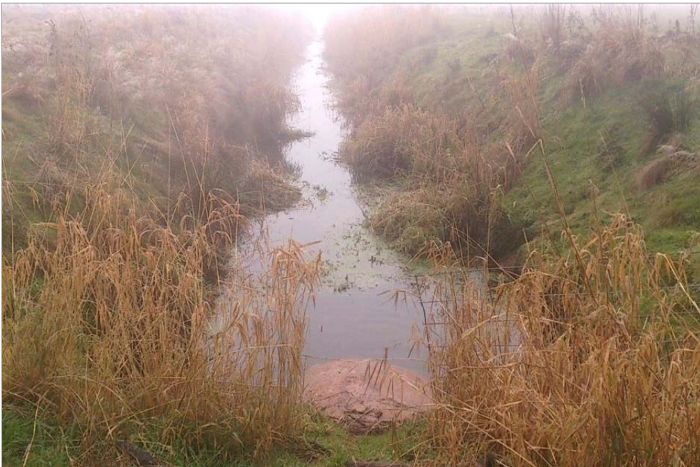
Figure 3: Spring channel ditch looking downstream with dense bank vegetation.
