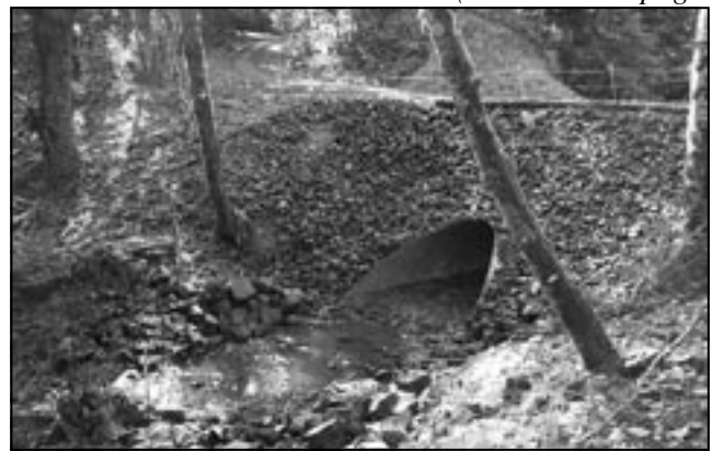
Perry Creek Post-Construction
