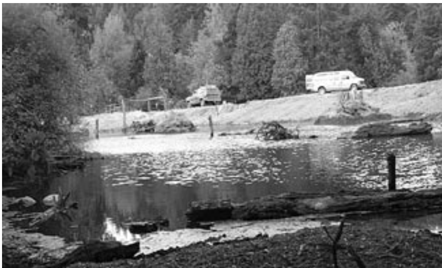
Lower Yelm Creek Post-Construction
