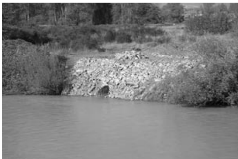
96th Street Oxbow Post-Construction
