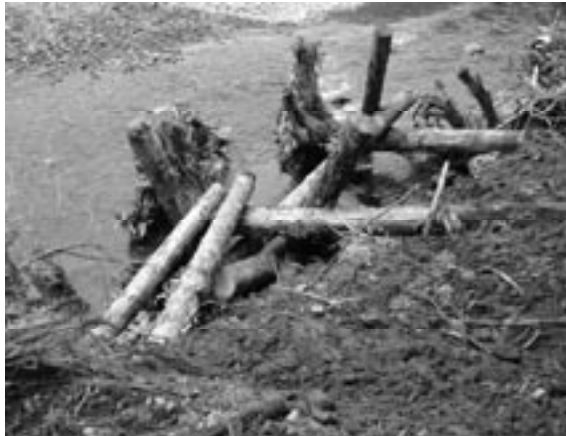
One of seven log jams placed on the Mashel
