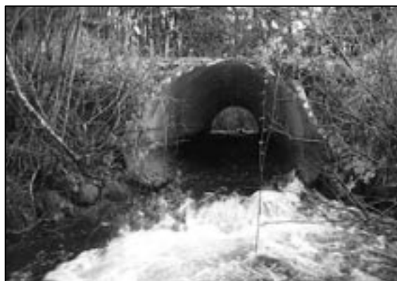
Eich Road Culvert Pre-Construction
