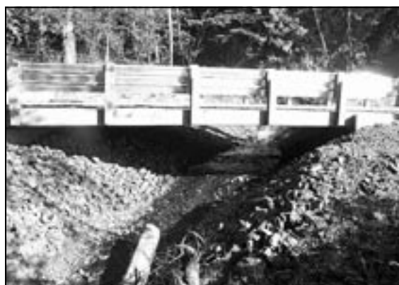
Eich Road Bridge Post- Construction
