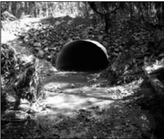
Perkins Creek Culvert Post-Construction
